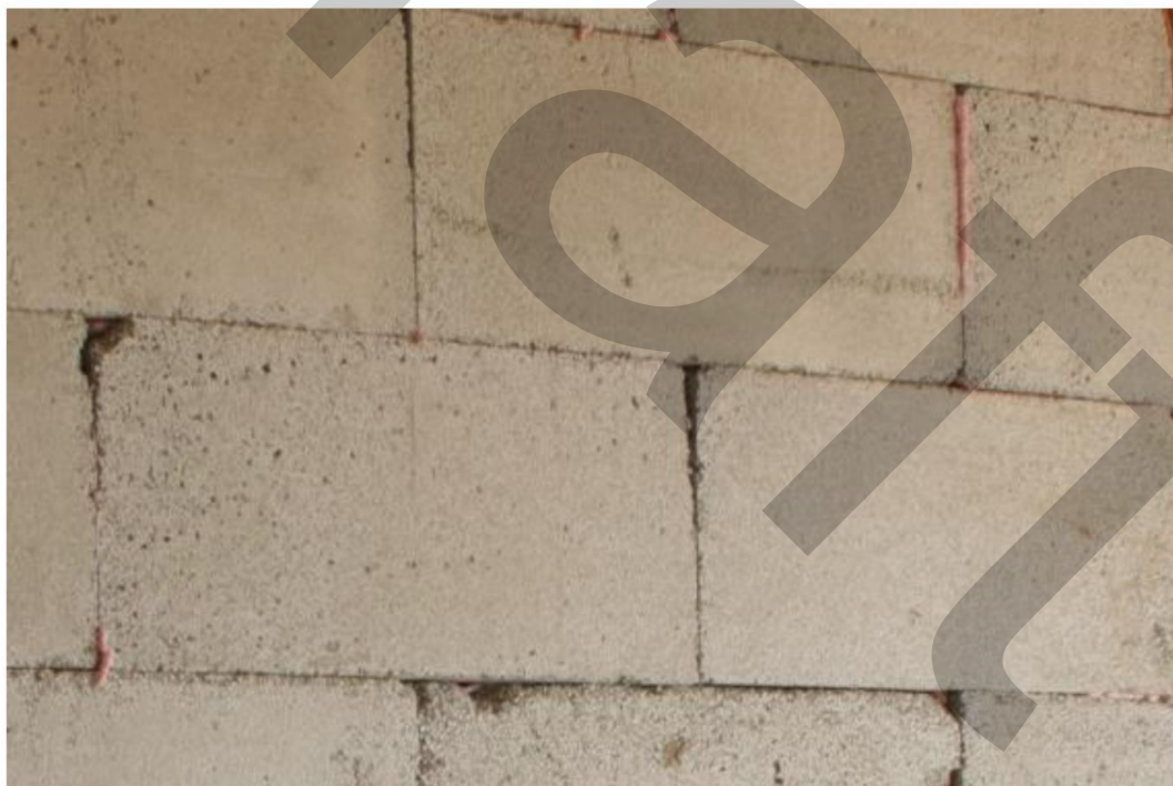
Figure 1f) Masonry unit made of lightweight concrete manufactured using polystyrene
